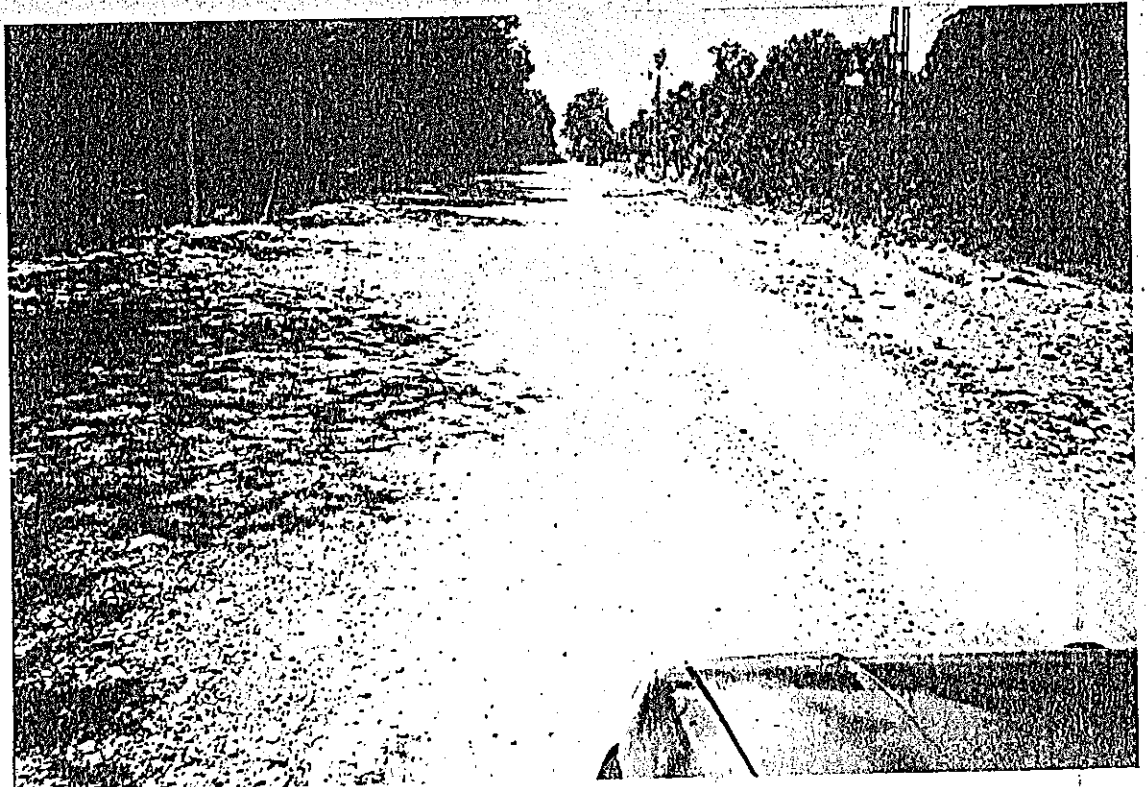
Fig. 5.1.5 Existing condition of the road surface after removal of Asphaltic Concrete surface.
