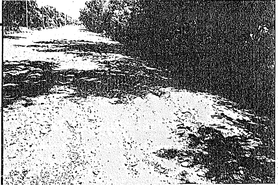
Fig. 5.1.4 At some locations, top of the base course layer has lost to some depth
