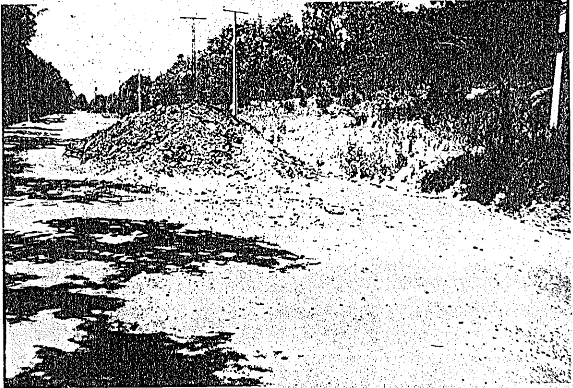
Fig. 5.1.2 Another site showing heap of asphaltic material
