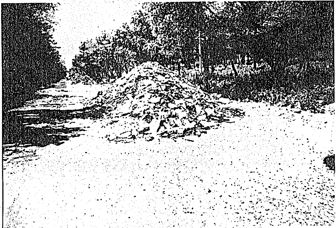
Fig. 5.1.1 Heap of Asphaltic binder and wearing course layers after removal by the bulldozer.
